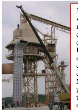
3. The new sections of duct were carefully lifted for installation. All dimensions were field checked by our Engineering Department to ensure that the new equipment would fit correctly. Our QC Manager inspected all parts to make sure that they measured to the customer's specifications.
