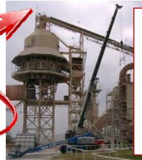
2. A downtime date was scheduled for the removal of the worn duct and the delivery and installation of the Technos replacement duct. This reduced the time and cost associated with repeated crane activities.
