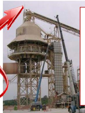
4. The new duct was put into place and installed as scheduled. All connections were matched and flanges bolted or welded to the existing sections. The customer was very pleased with the result. Another Technos project successfully completed!
